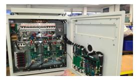
The chargers consist of an input automatic changeover switch, an auto transformer, rectifier modules, and output distribution
