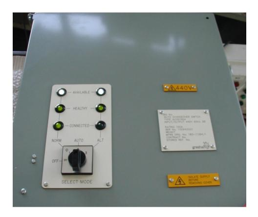
The Automatic changeover switch (ACOS) provide the capability to automatically switch a load between a 'Normal' and an 'Alternative' supply. Switching employs mechanically interlocked contactors and is controlled by electronic monitoring of the supply. Override facilities are provided which allow for manual selection of either power source.
