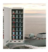
Valve regulated lead acid batteries are used to support ships essential DC supplies via output circuit breakers.
