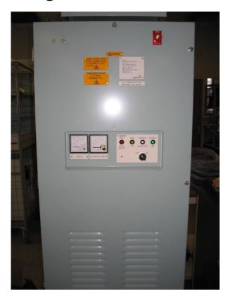
The Transformer Rectifier Unit 3RC10kF is intended for shipboard Helicopter Start applications. There are three basic modes of operation
